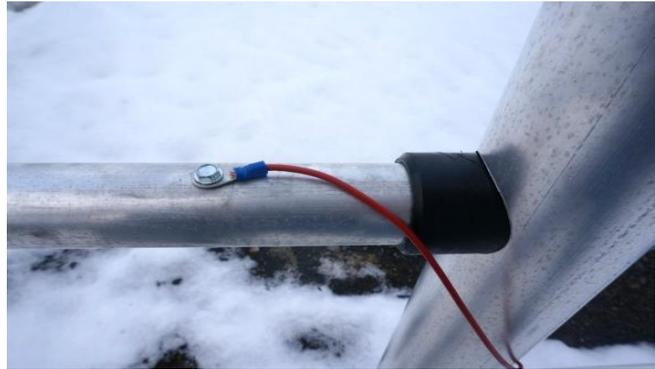
Connect the energizer to each rail level. Ensure the solid connection of energizer for example with a cable lug and a screw.
