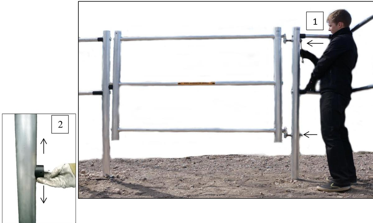
Place the hinges to the gateposts (1). Place the support part of the gate (2) with 10 mm socket wrench.
